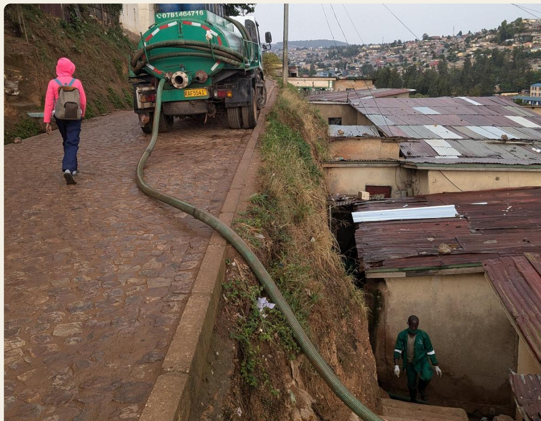
Steep hills: many pits sit far below the road
